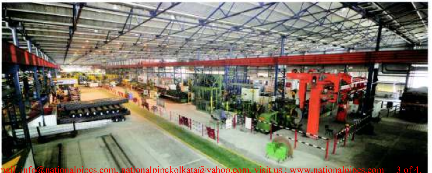
Tubes being manufactured in state-of-the-art HFW Mill
